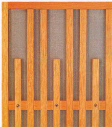
A unifying theme. Latticework is used on all of the cabinet doors. Some intersecting members are pinned using brass, colored an antique brown.
