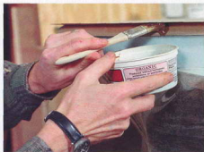
After the first pressing, the edge is prepared for gluing. First, spread plastic resin glue around the edge and deep into the crevice.
